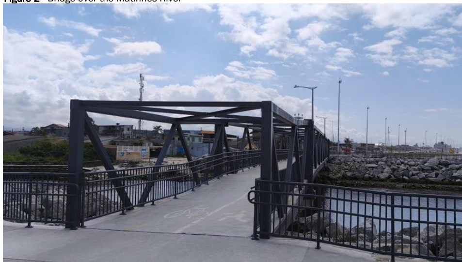
Figure 2 - Bridge over the Matinhos River
